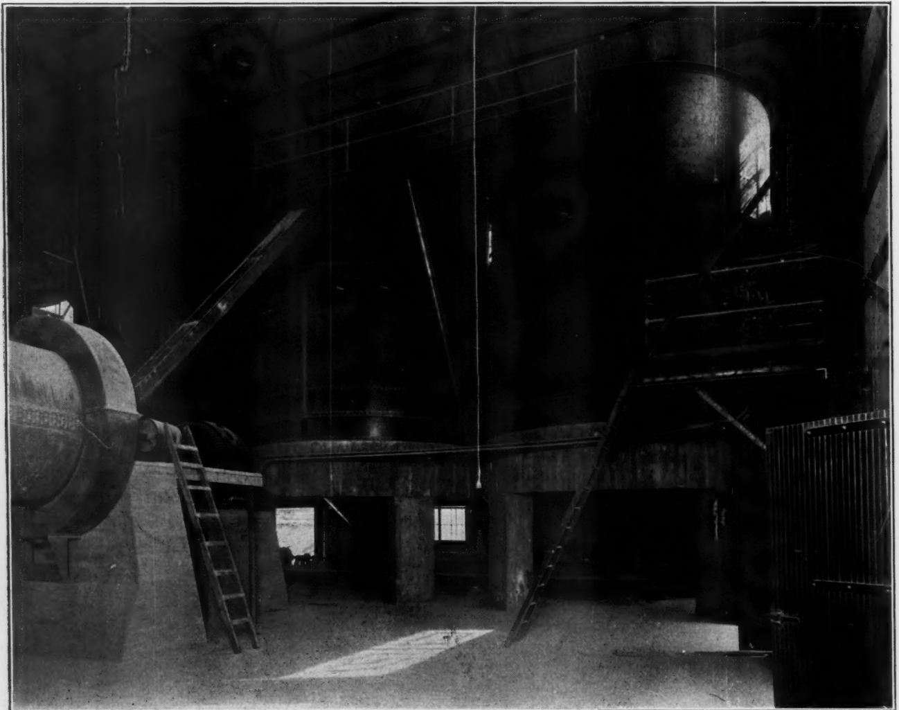
View of Large Steel Tanks Where Brixment is Treated to Make it Extremely Plastic.
